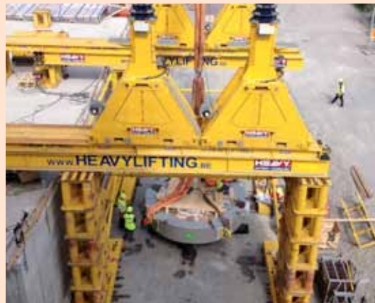
The cyclotron was hoisted into the Skandionklinik in spring 2013 – an important milestone on the journey to the first treatment in 2015.
